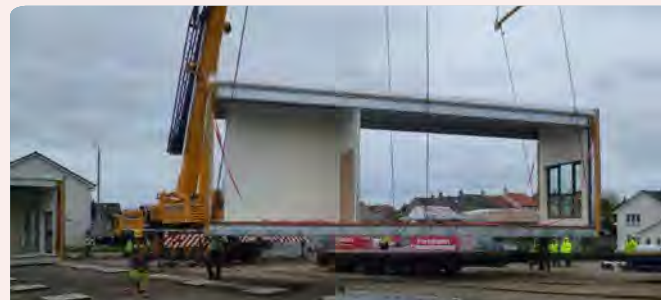
Lynburn Primary School Nursery, Dunfermline, Fife - construction
