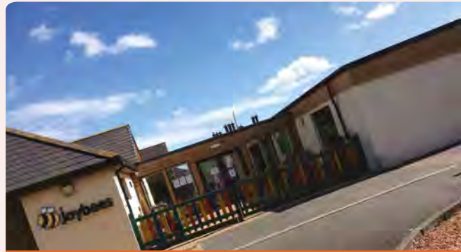
Original accommodation links to renovated workshop
