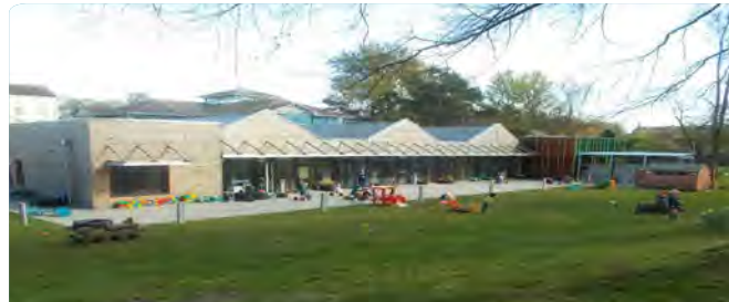
Rocking Horse nursery, Aberdeen (BMJ Architects)
