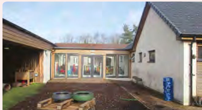
Corridor linking both buildings
