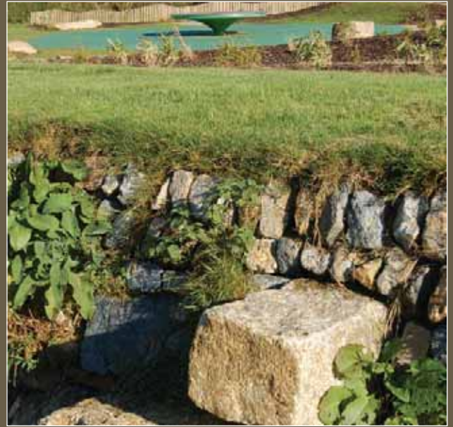
Projecting 'climbable' steps in the dry-stone wall.
